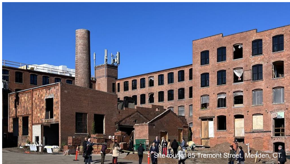
Existing conditions image of 85 Tremont Street site today.
